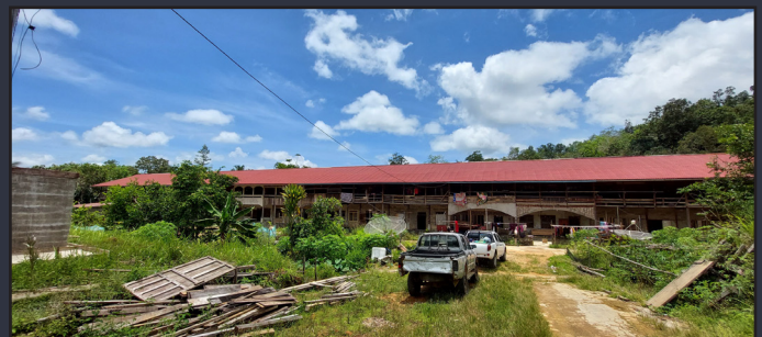
Longhouse 'Rumah Betang' of Iban community in Sungai Luar hamlet, Sungai Abau Village. The team stayed here with the residents and conducted various participatory activities.
